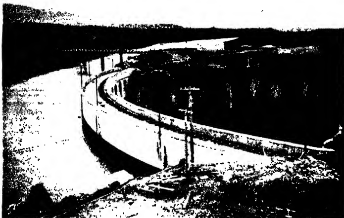
FIG. 145. THE ARAPUNI DAM
